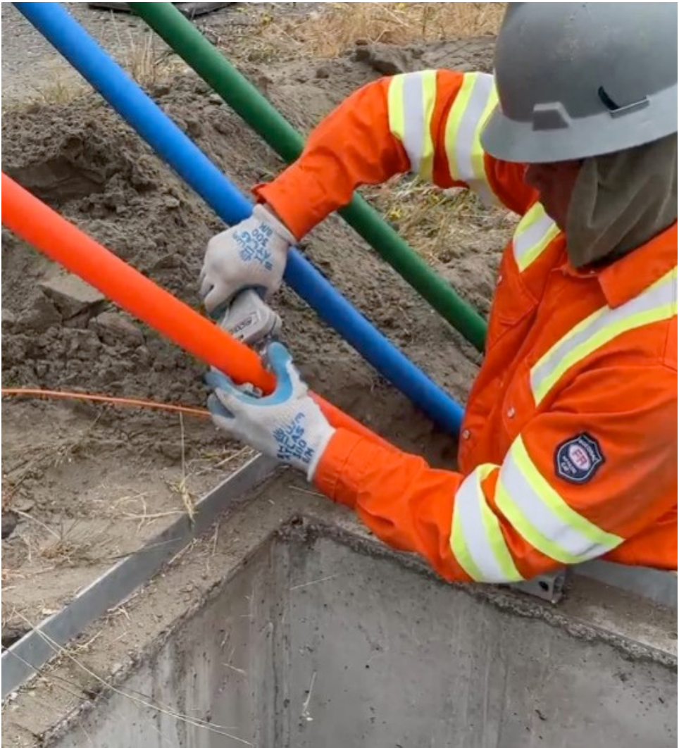
Installation of conduit the protective structure for the broadband fiber.
